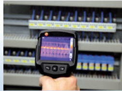
Check electrical installations
