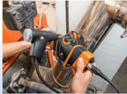
Efficient adjustment of heating systems
